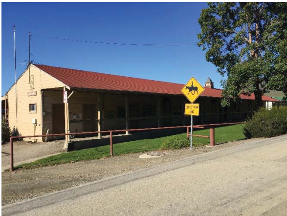
Photo #21 Additional horse stables west of EHS, facing north.
