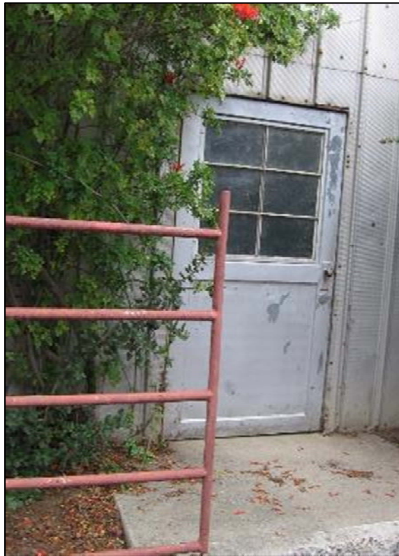
Figure 57. Original steel door with 6-light fixed glazing on west elevation near southwest corner, Beef Unit.
