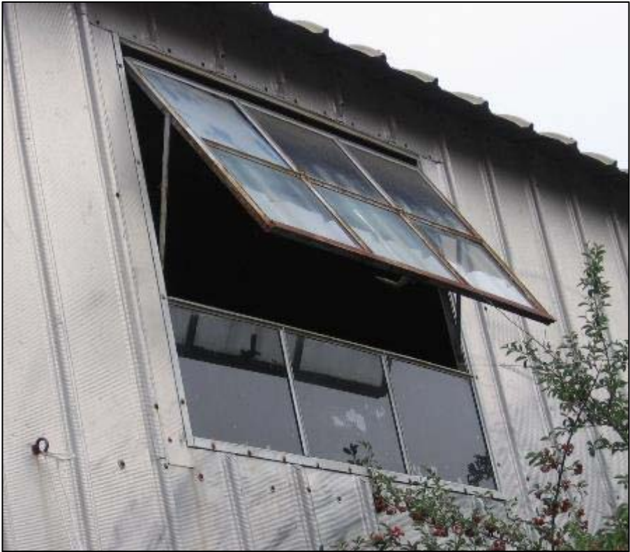
Figure 49. All of the windows are two-part steel sash; the upper 6-light sash is awning mounted, and the lower sash has 3 fixed lights.
