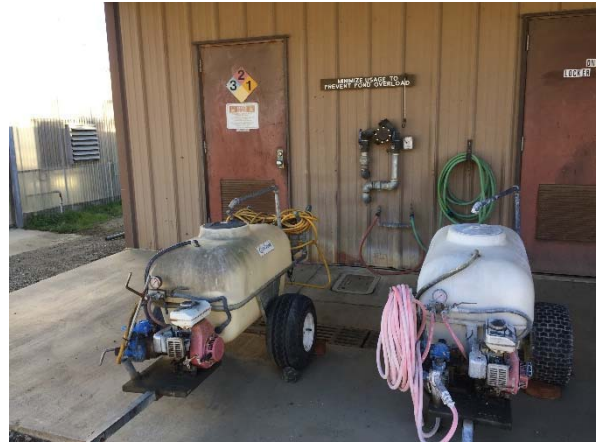
Photo #2 View of the chemical mixing area and floor drain at EHS Building 048-M, facing south.
