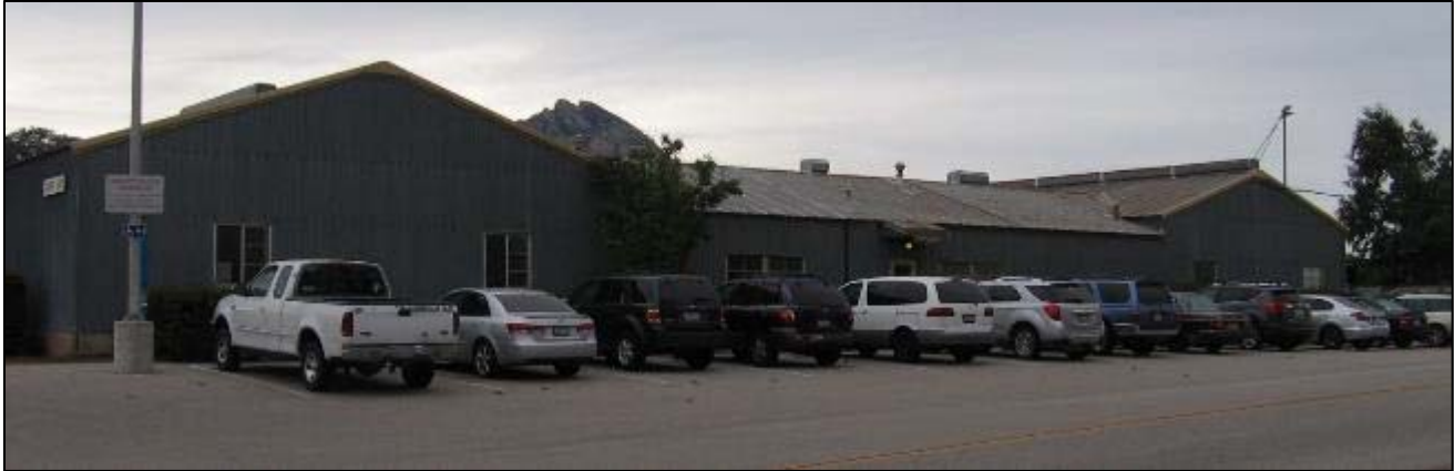
Figure 70. Northeast elevation of main Crop Science building.
