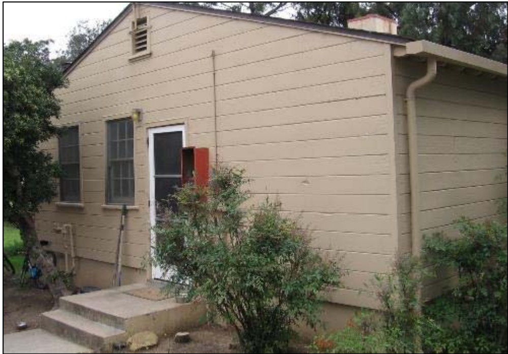
Figure 46. North elevation, Beef Unit Herdsman Residence.
