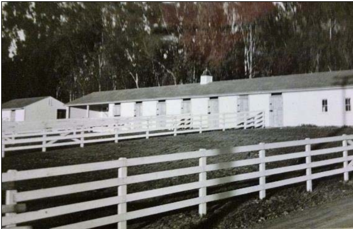
Figure 4. East elevation of Mare Barn and paddocks at their original location (University Archives).
