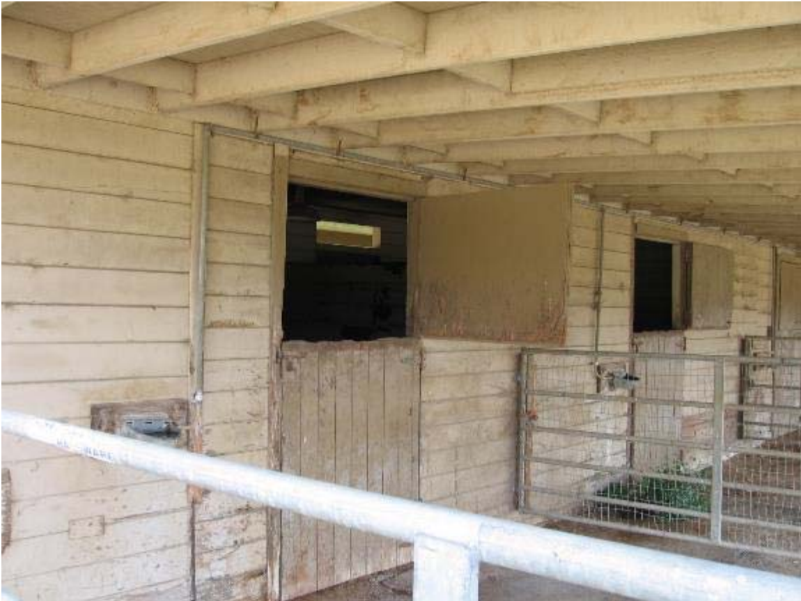
Figure 29. West elevation, stall doors leading into paddocks sheltered under shed-roof addition, Mare Barn.
