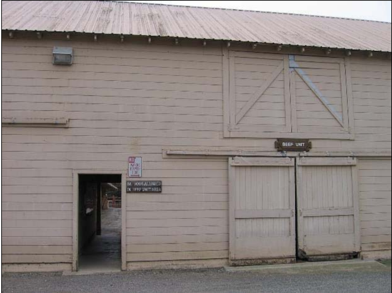
Figure 59. Principal (north) elevation of barn, showing passageway to feeding stalls and two types of barn doors, Beef Unit Feed Unit.
