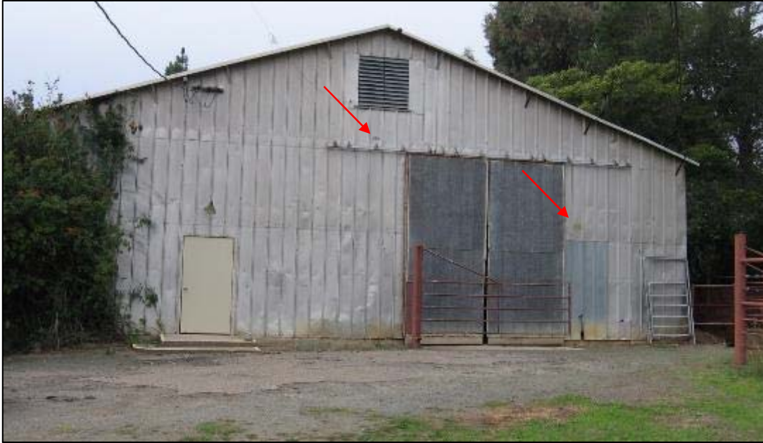
Figure 50. East elevation, Beef Unit. The arrows indicate the location of the two Butler building plaques.
