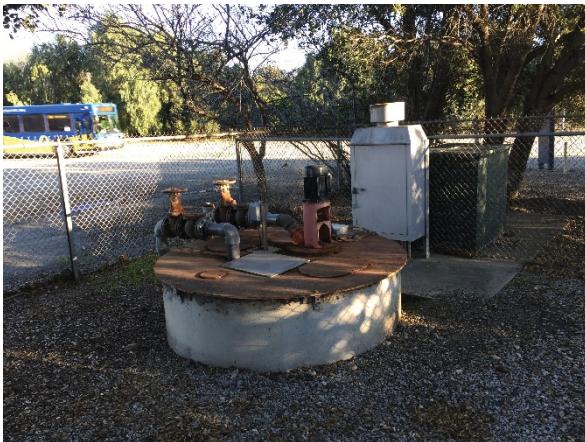
Photo #27 Pump station at the southern portion of the CU, facing south.
