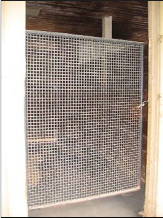
Figure 33. One of the original Mare Barn welded gates, made by students in the School's Metal Shop.
