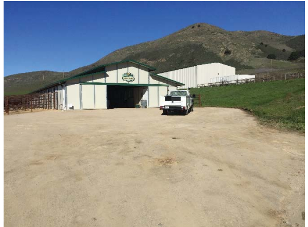
Photo #20 View of horse stables north of EHS, facing north.
