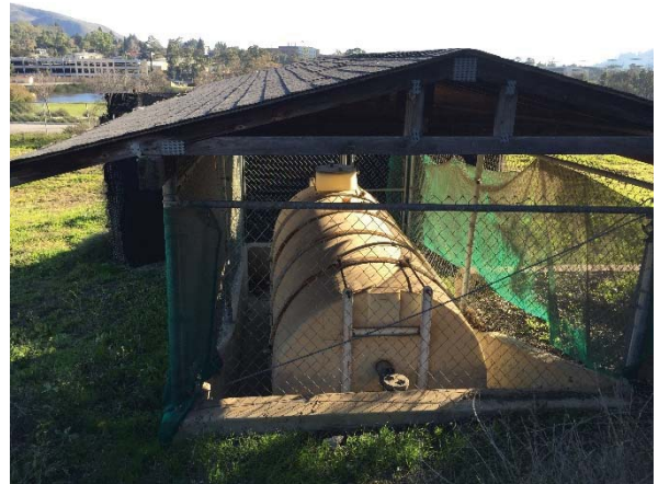
Photo #8 View the pesticide tank south of Building 048-M, facing south.
