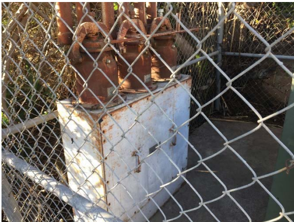
Photo #15 View of the PCB-containing oil filled cutout (OFC) switch at the south end of the EHS buildings, facing north.
