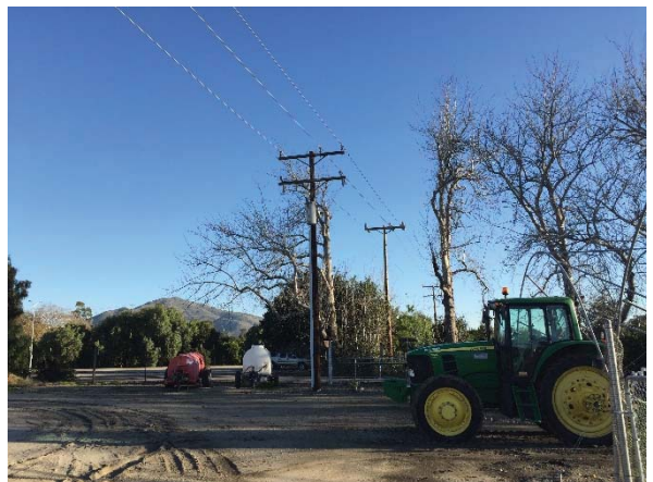
Photo #24 View of tracker storage and a pole-mounted transformer at the CU, facing east.
