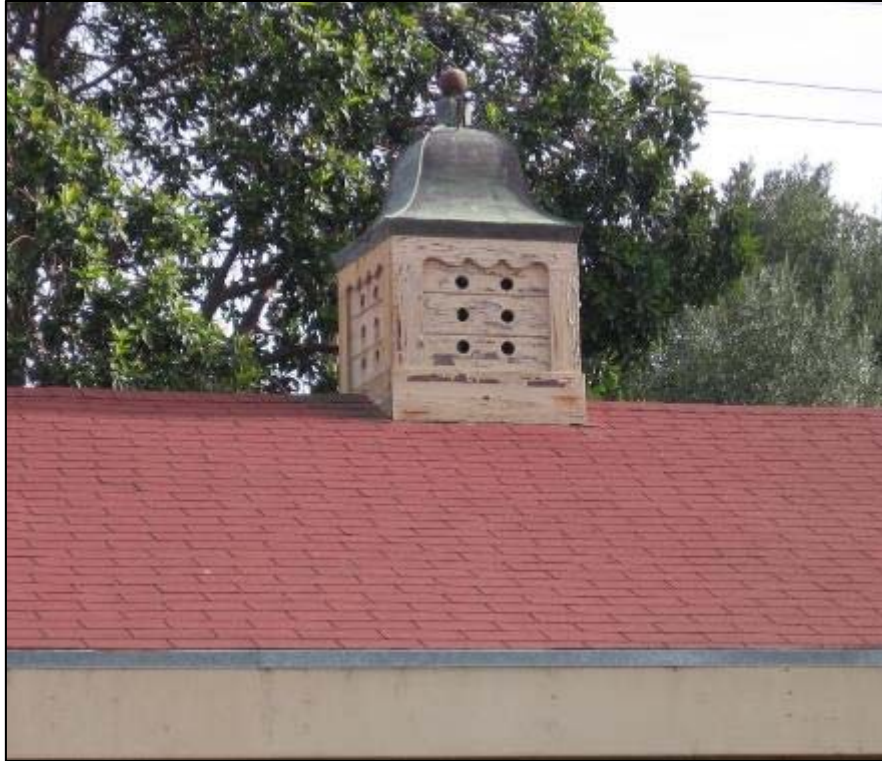
Figure 34. Original cupola with metal sheathing made by students in the School's Metal Shop. The cupola was Bartges' way of distinguishing the building as a barn for Thoroughbreds.
