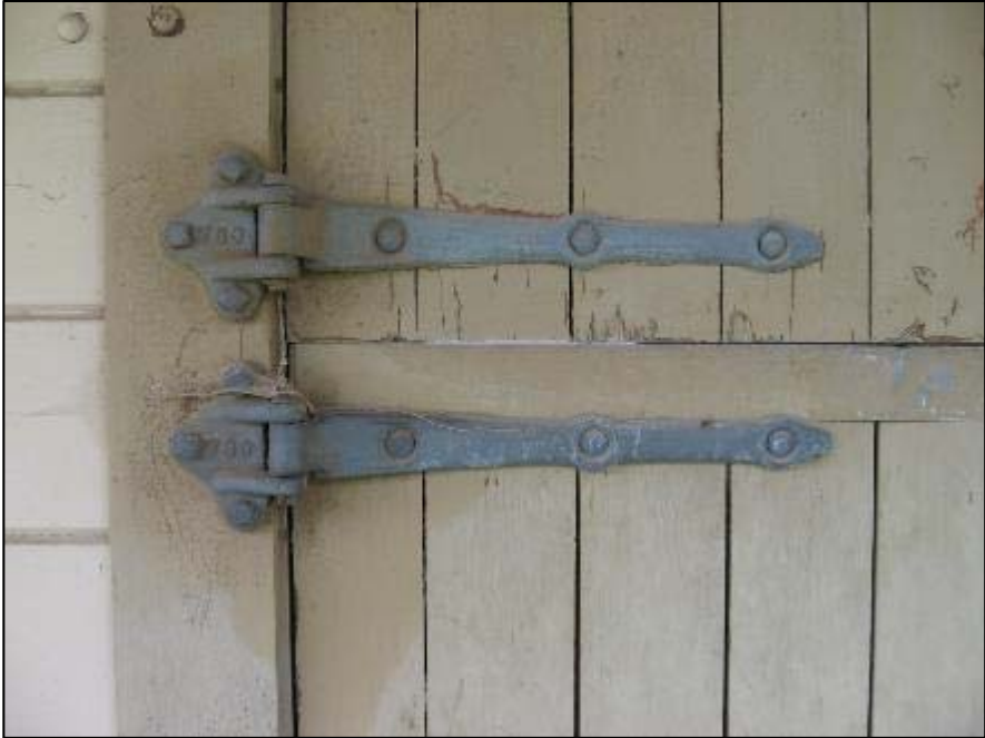
Figure 32. Original strap hinges on corridor stall doors, Mare Barn.
