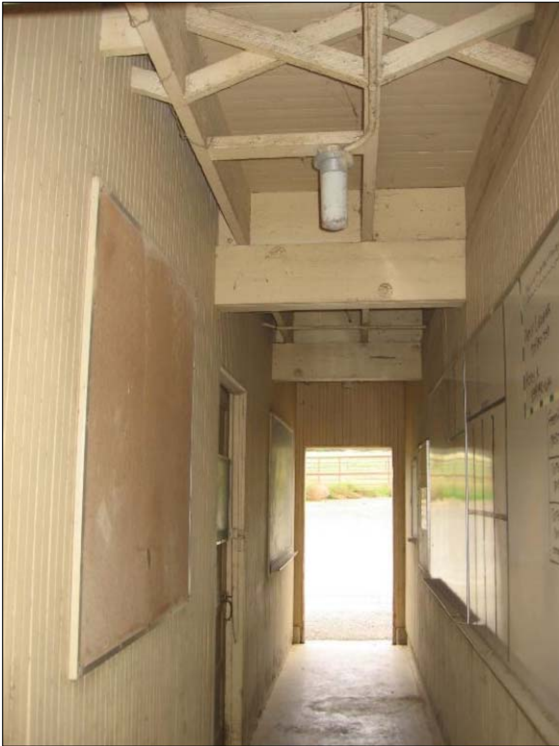
Figure 60. Interior of passageway through barn to feeding stalls, Beef Unit Feed Unit. Walls are clad in bead board. Cross bracing at ceiling supports joists for second floor.
