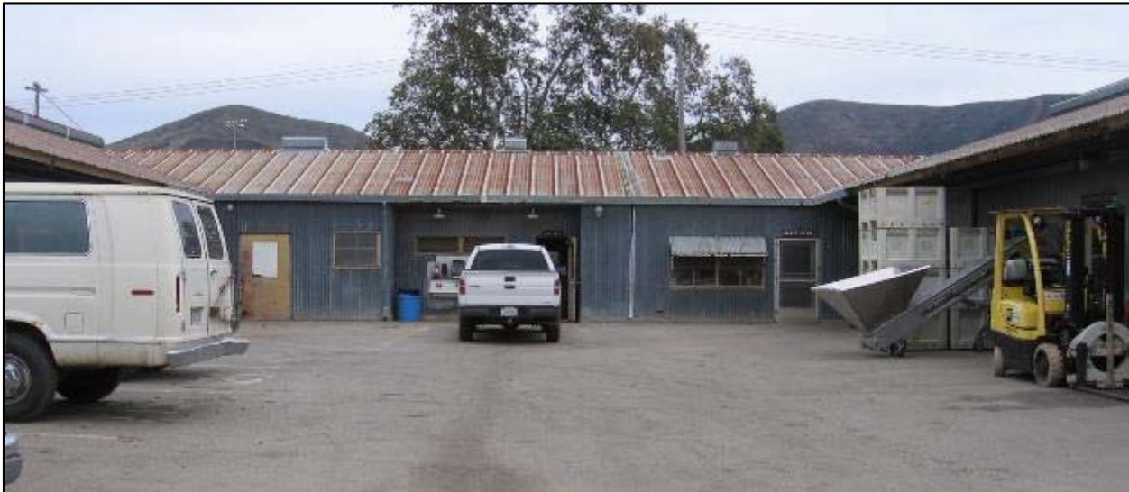
Figure 65. Interior yard on west side of U-shaped Crop Science building.
