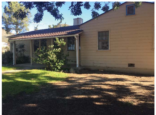
Photo #30 Front of the residence near the Beef Unit, facing northeast.
