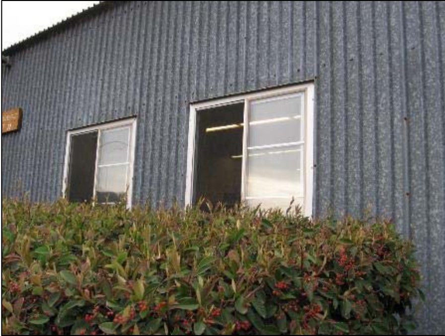
Figure 68. Southeast elevation with replacement windows, main Crop Science building.
