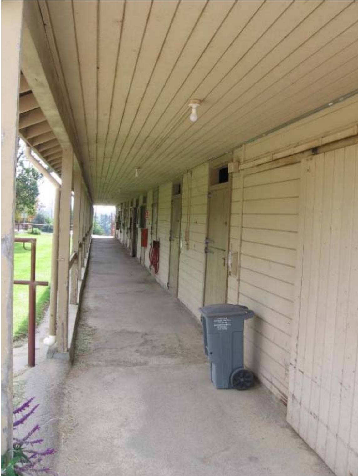
Figure 27. View of corridor on east elevation, looking south, Mare Barn.
