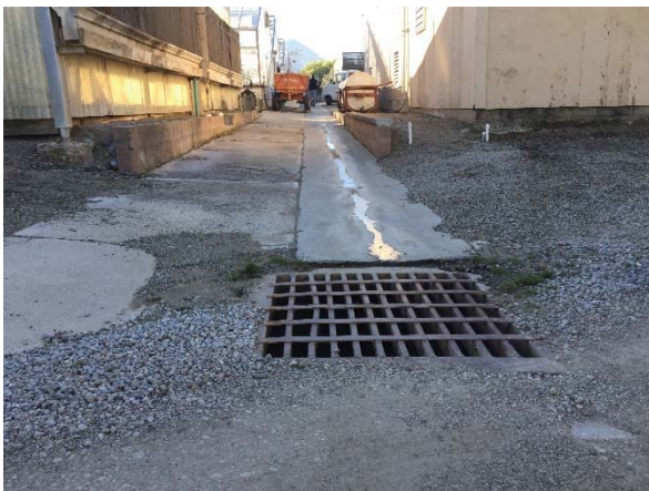
Photo #17 View of a storm water drain at EHS, facing west.
