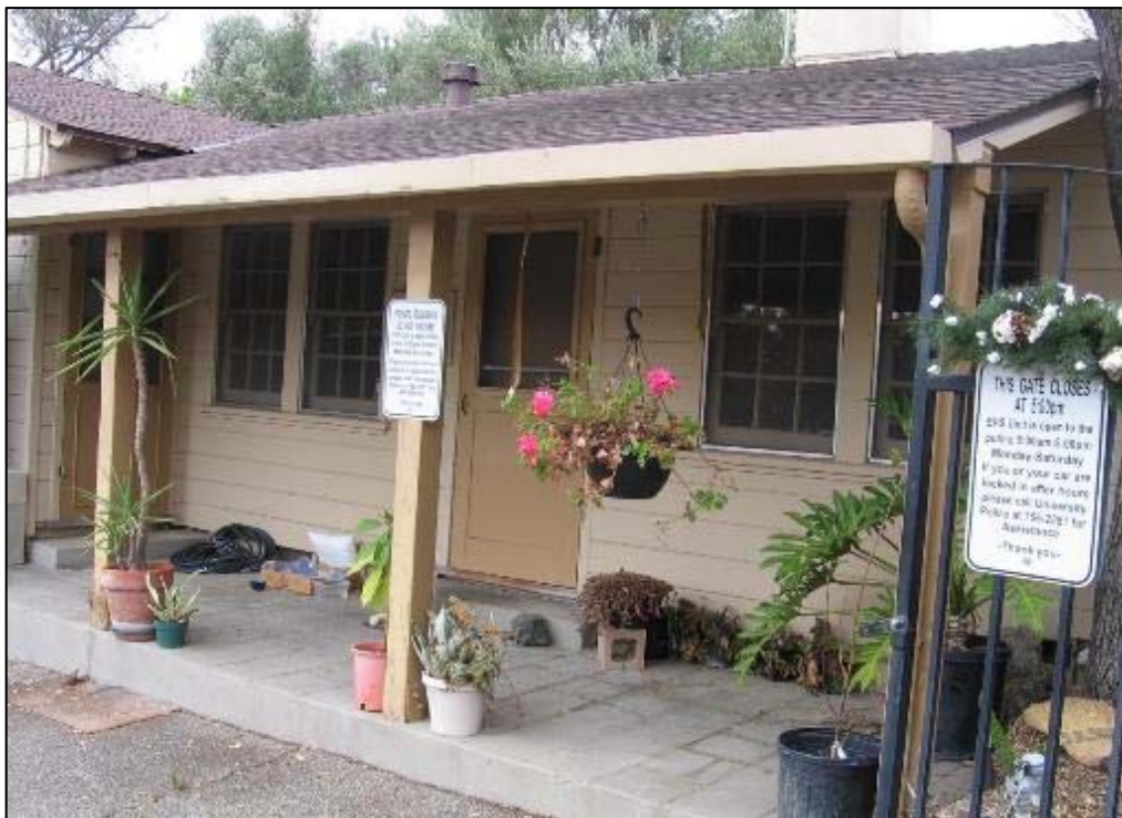
Figure 36. East end of south elevation, Environmental Horticulture Science Residence.
