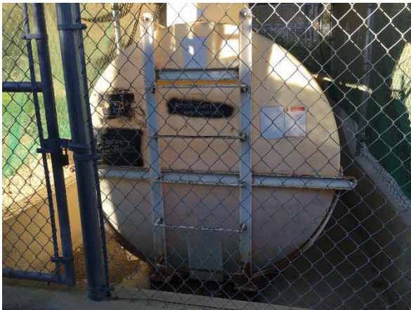
Photo #9 View the pesticide tank south of Building 048-M, facing north.
