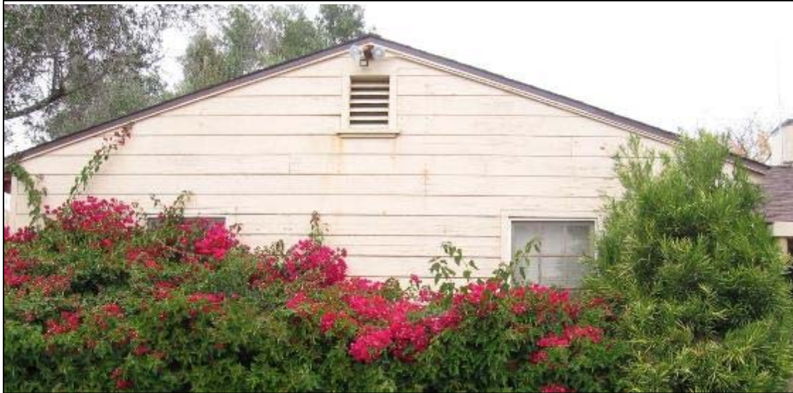
Figure 35. West end of south elevation, Environmental Horticulture Science Residence.
