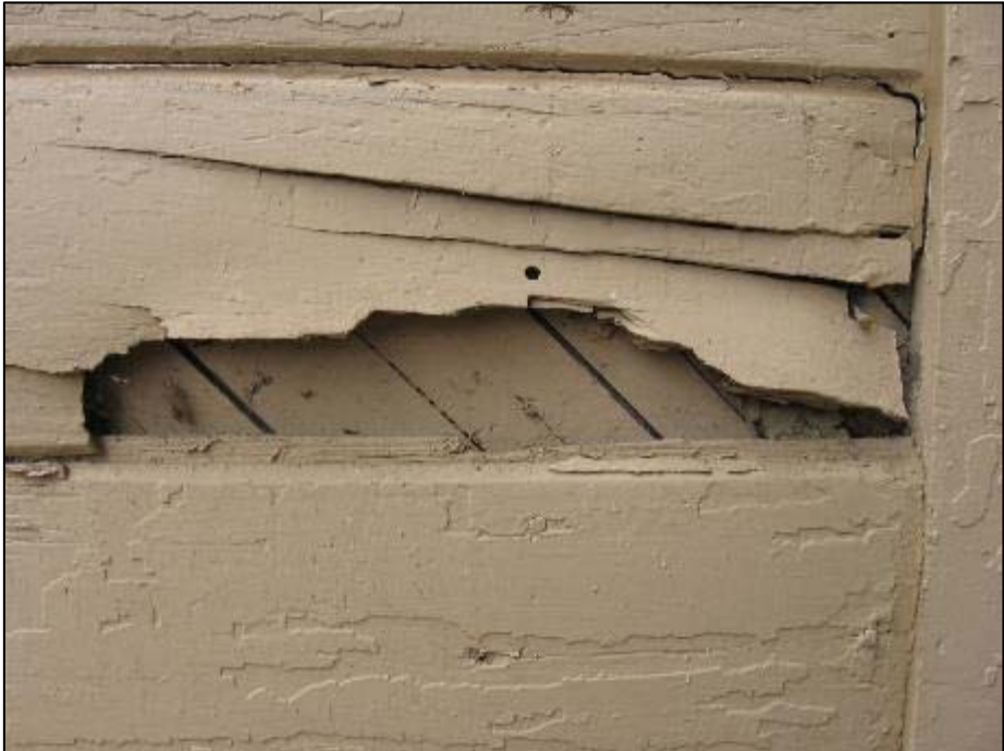
Figure 44. Damaged V-groove rustic siding at southeast corner, Beef Unit Herdsman Residence, revealing double-wall construction.
