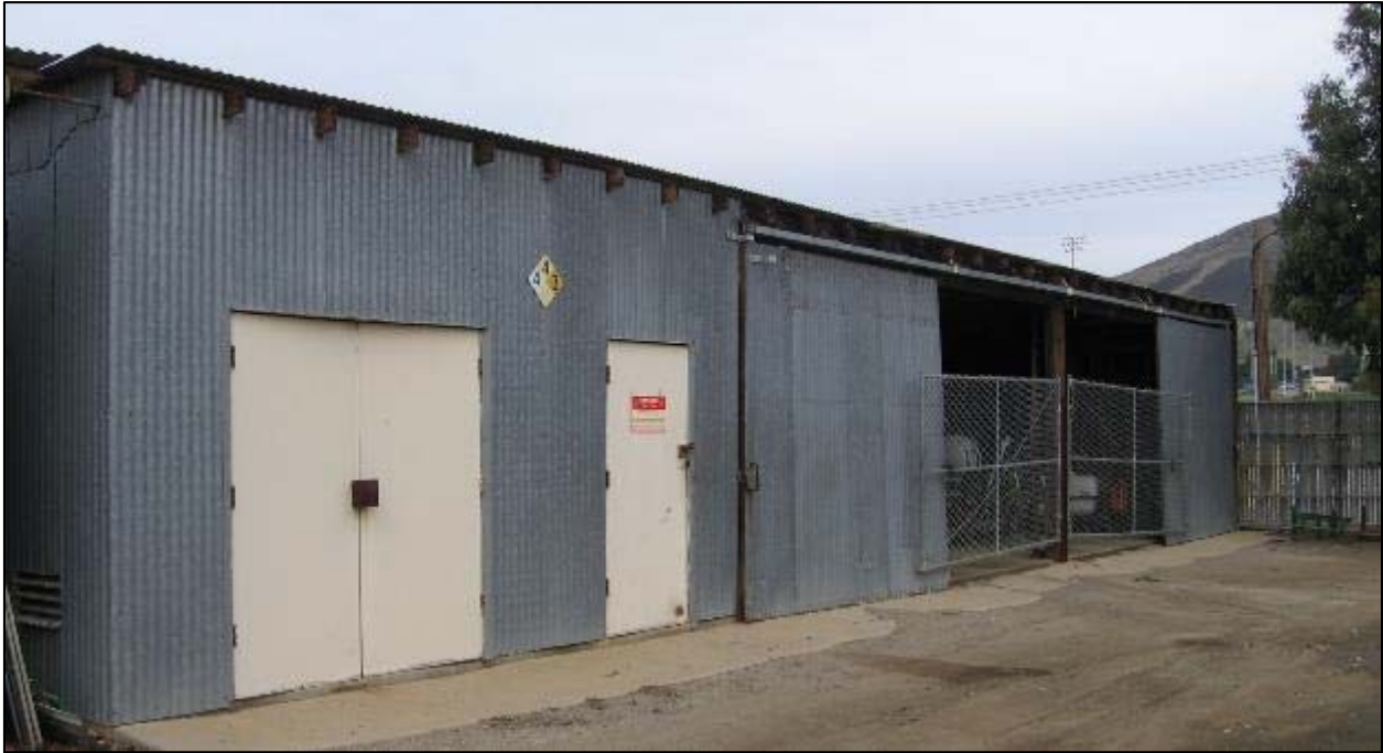
Figure 74. Storage sheds to the right of the Irrigation Pipe Storage Shed.
