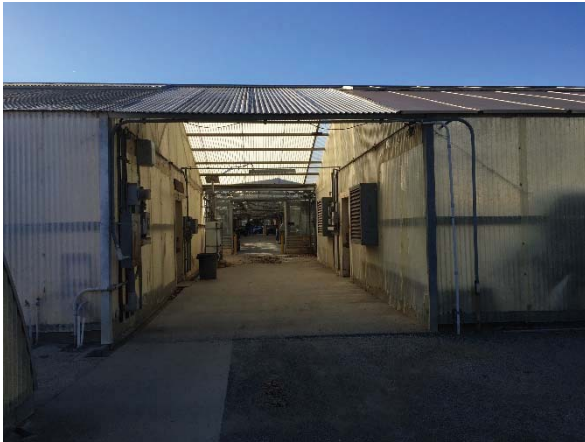
Photo #1 View of the Environmental Horticultural Science (EHS) building entrance, facing east.
