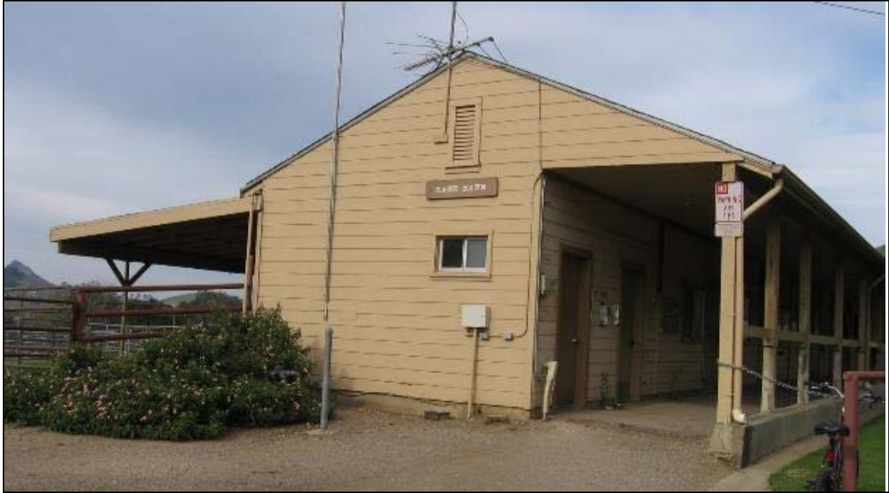
Figure 30. South gable end, showing roof articulation, Mare Barn.
