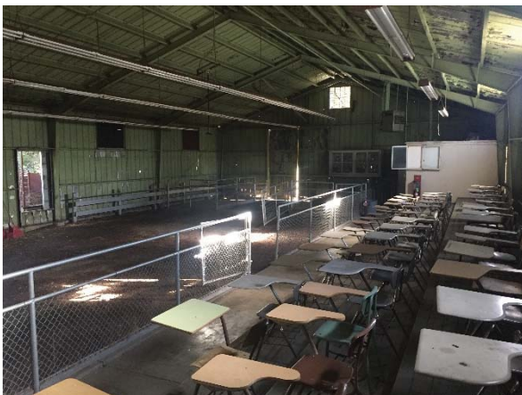
Photo #29 Inside of the Agricultural Pavilion, facing northeast.
