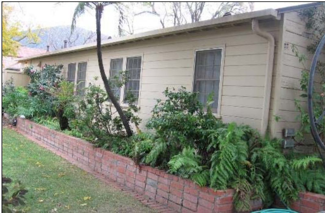
Figure 38. North (rear) elevation, Environmental Horticulture Science Residence, with raised stacked brick planting bed.
