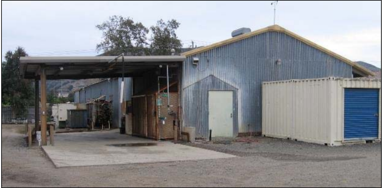
Figure 66. West corner of main Crop Science building.
