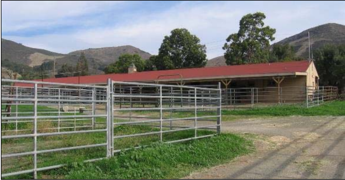
Figure 28. West elevation, Mare Barn.
