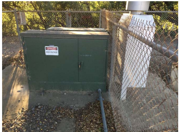
Photo #28 Pad-mounted transformer south of the pump station, facing west.
